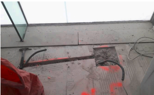
Chiseling out of cable ducts
