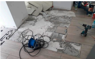
Demolition (floor tiles)
